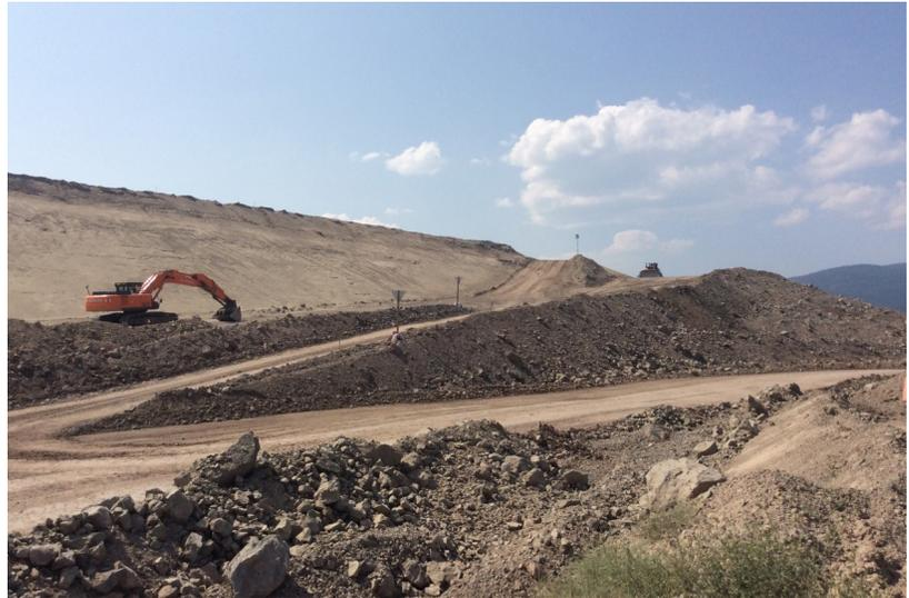
By the end of 2018, waste rock will make up more than half of the material used in tailings dam construction, or roughly 800,000 cubic metres. In the months and years ahead, New Afton will work to continually maximize sand production while incorporating more and more recovered waste rock as crews continue to prioritize safety and high-quality construction.
